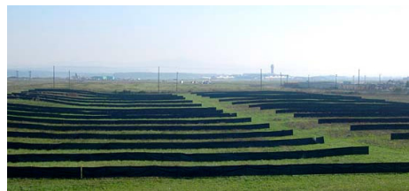
Construction silt fencing breaks up the line of sight in large open areas. This decreases visibility for geese, when their visibility is limited, the geese sense a predator may be waiting beyond the obstruction.
